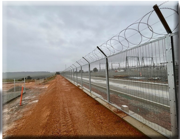
2400mm high Anti Climb 358 high security fencing completed by KFW WA for Scee on the Collie Bess Transformer Project
